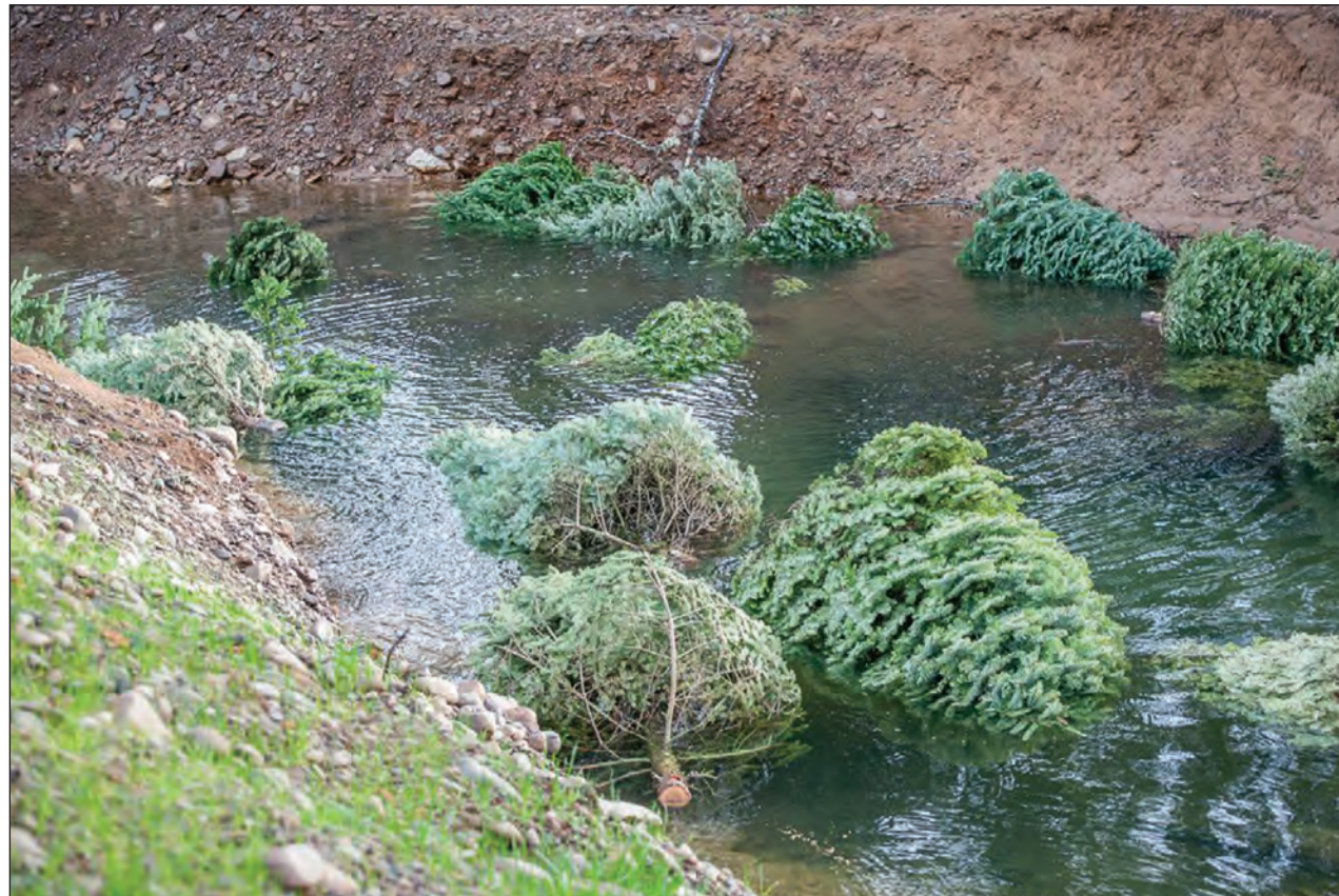
TREES FOR TROUT: Trout Unlimited and RI DEM team up to help control water flow in rivers and erosion through the strategic placement of Christmas trees. (Submitted photo)
